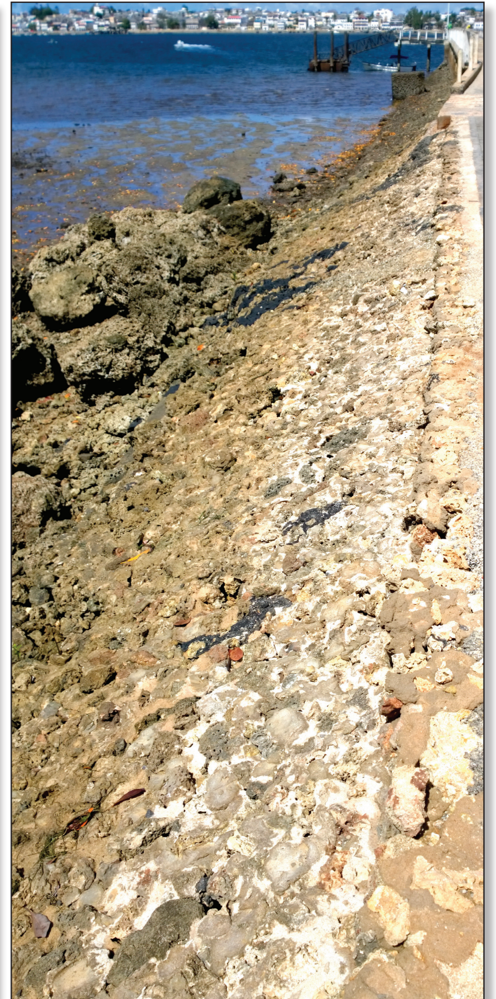
Figure 25: Photograph taken from point P (2) - jetty at airport
