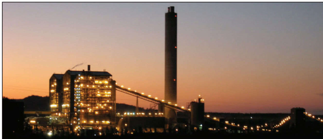
Figure 3: Example of a power plant at night
