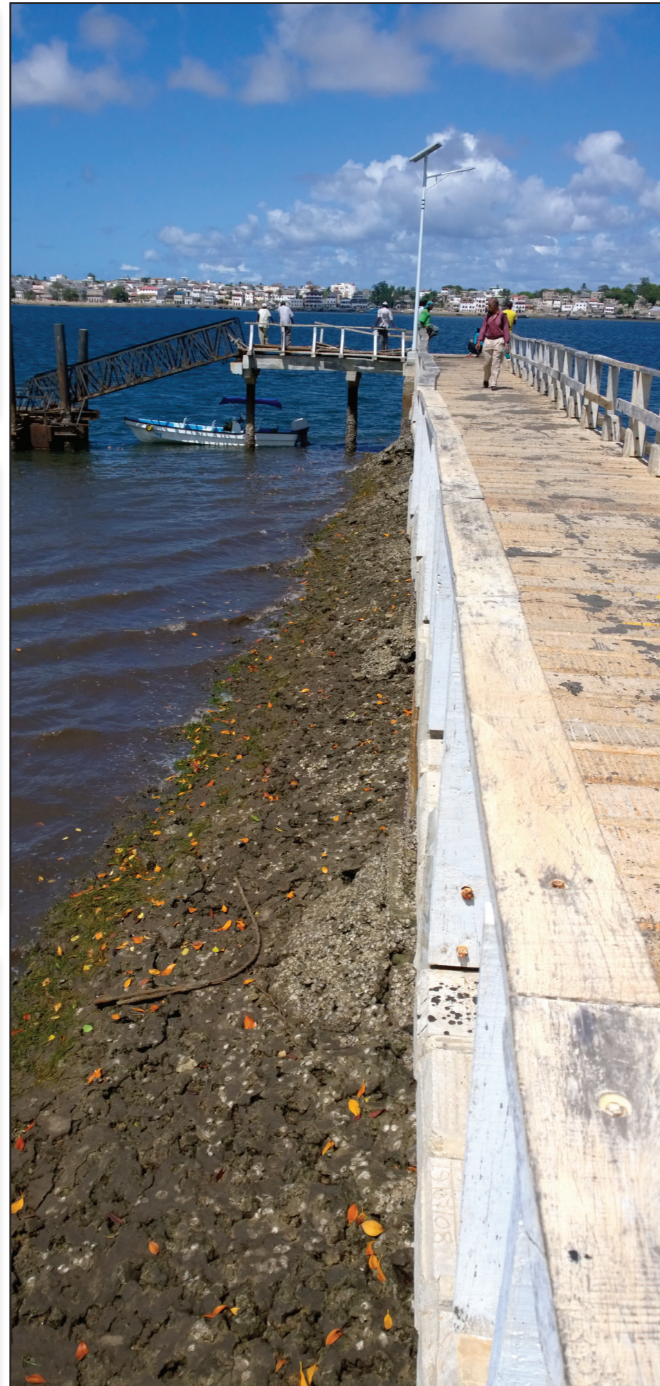
Figure 24: Photograph taken from point P (1) - jetty at airport
