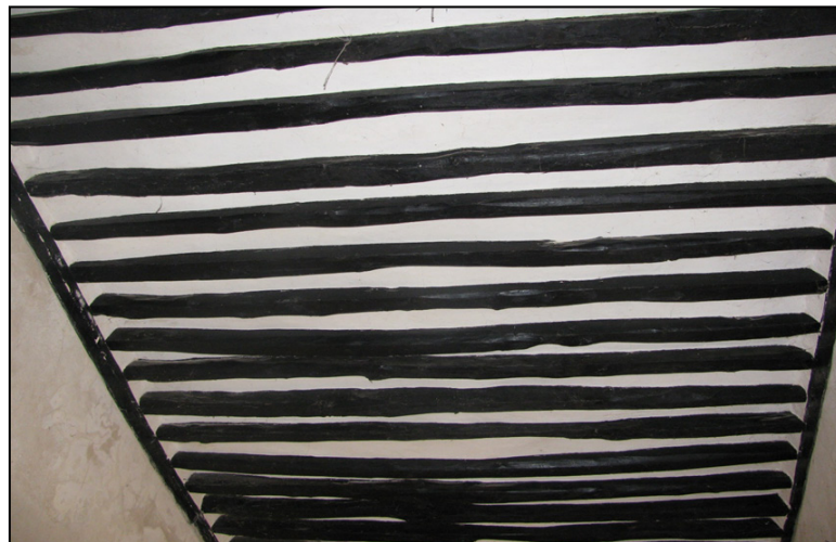
Figure 8-23: Example of a ceiling made from Mangrove timber
