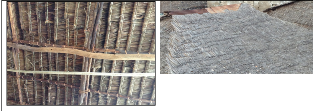
Figure 8-24: Roof and thatch supported by Mangrove poles
