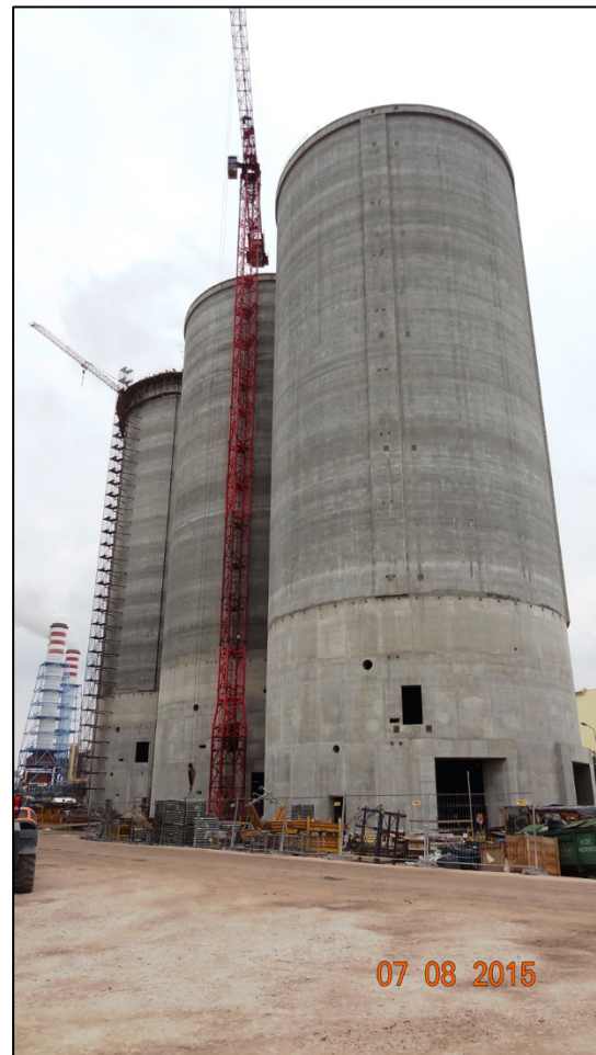
Figure 4-10: Fly ash silos under construction
