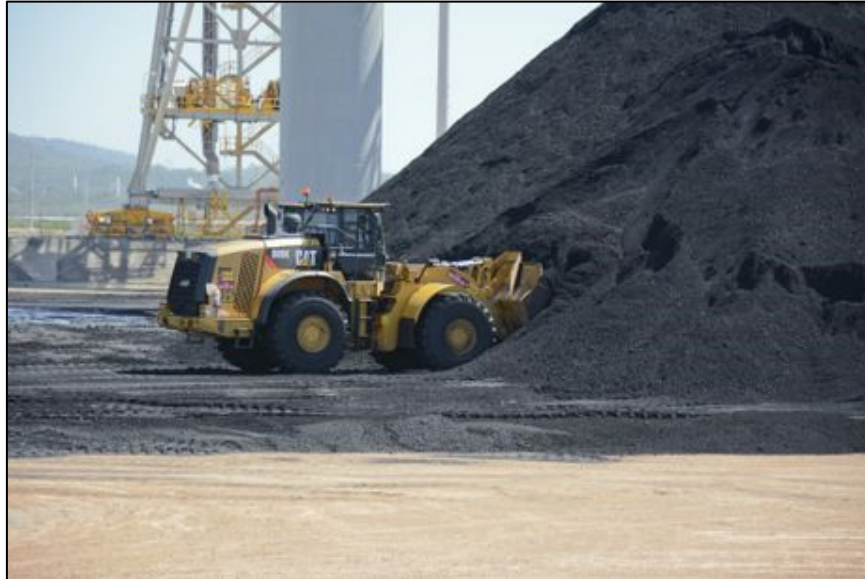
Figure 4-7: Front end wheel loader in operation within a coal stock yard
